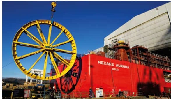
Positioning the lay wheel for the 'Nexans Aurora' CLV vessel.
