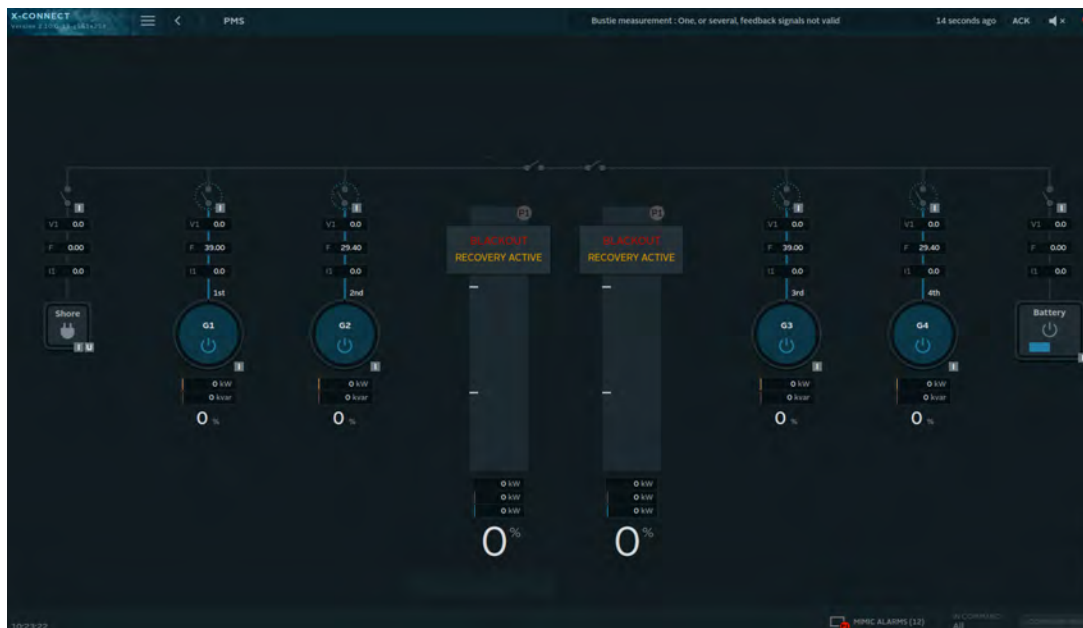
Figure 8: ULSTEIN PMS™ is performing blackout recovery
